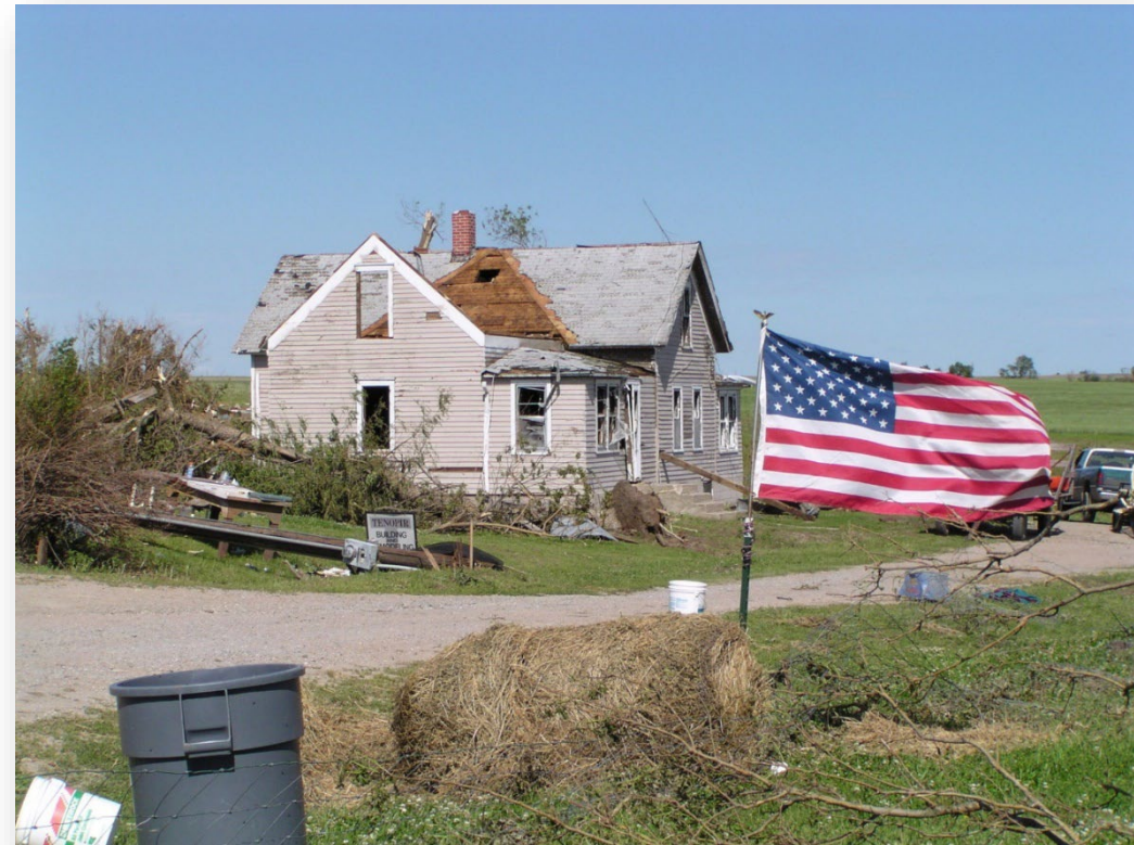
Farm near Wilber, Nebraska damaged by a tornado, S. Cochran (2004)
